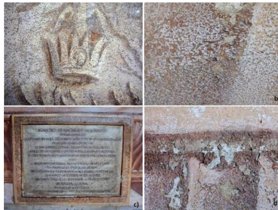
Fig. 2. Degradation phenomena on the funerary monument: a) surface with black spots; b) film-white paint; c) tombstone; d) deficiencies, lifting the film.
